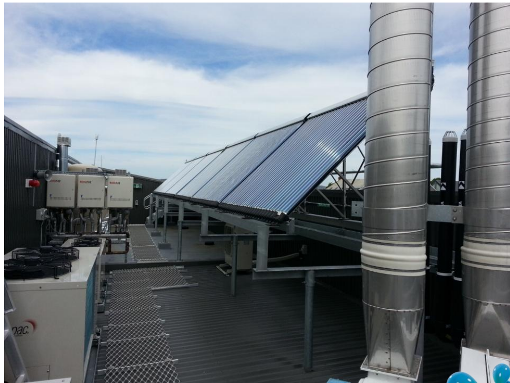
Gas boosted solar hot water system
