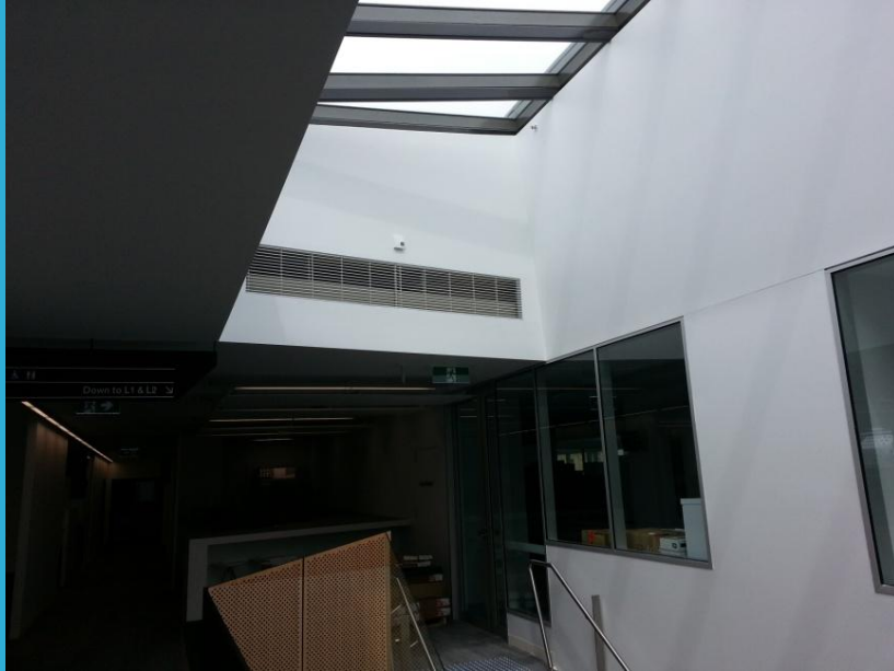
Internal skylight & ventilation inlet
